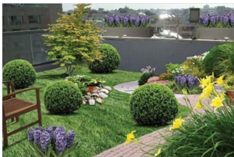
Figure 4. Intensive green roof
