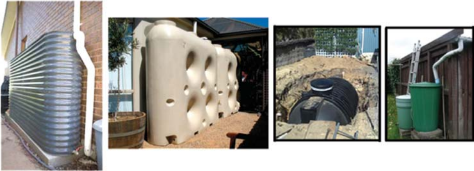
Figure 7. Tanks for rain harvesting
